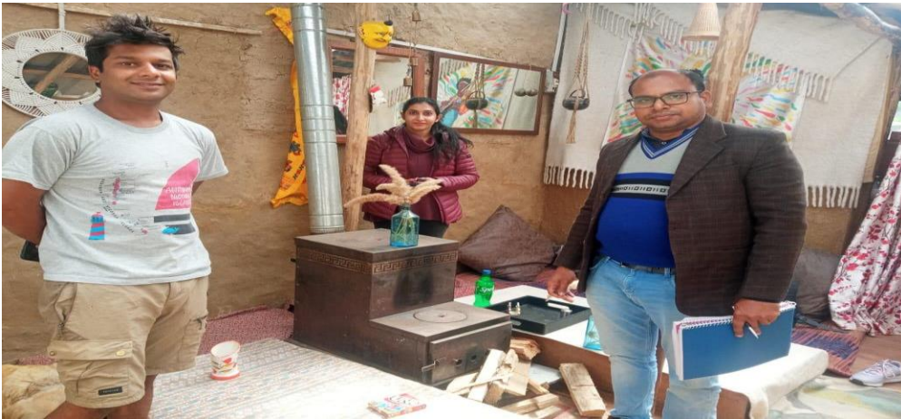
HRS Stove (Eco 1) installed in homestay in Himachal Pradesh.
