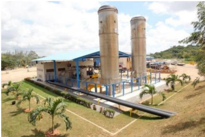
Landfill Gas flaring plant installed at CTR Candeias in 2015
