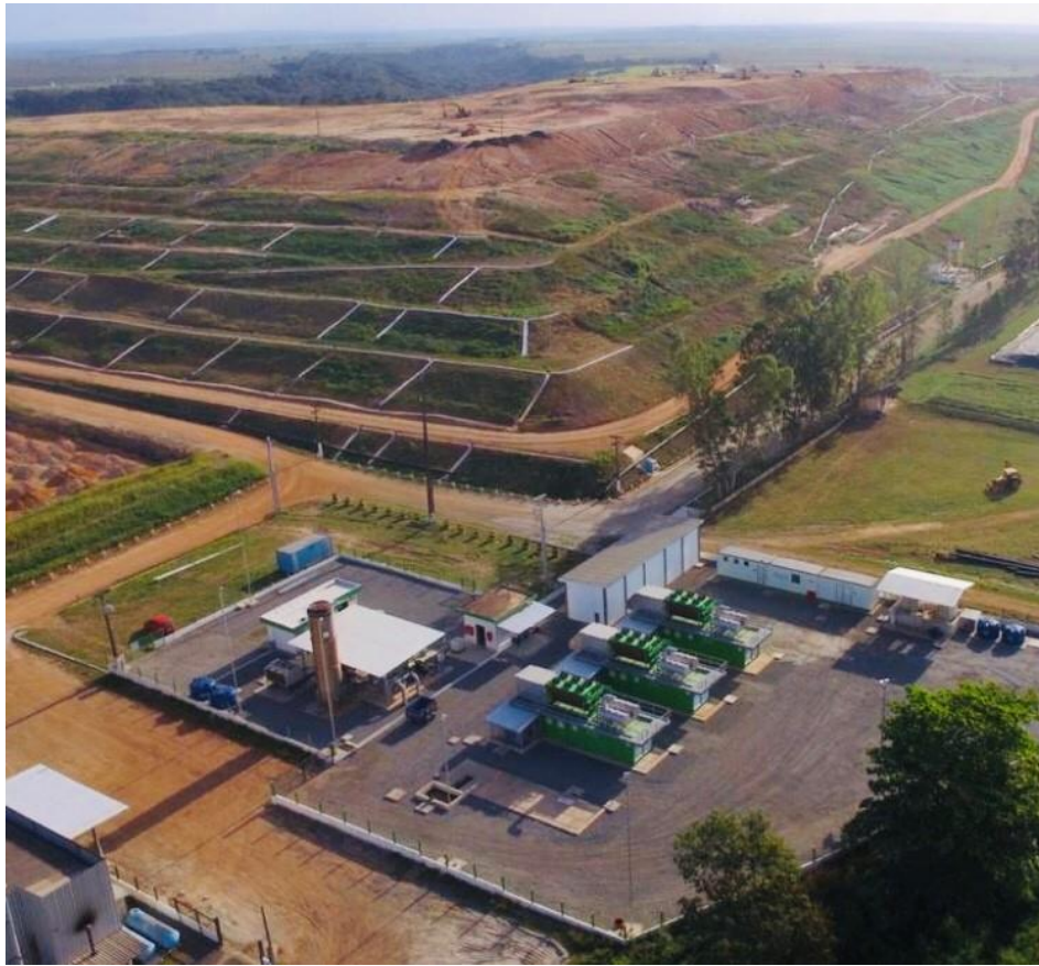
Aerial view of the LFG plant, March 2021
